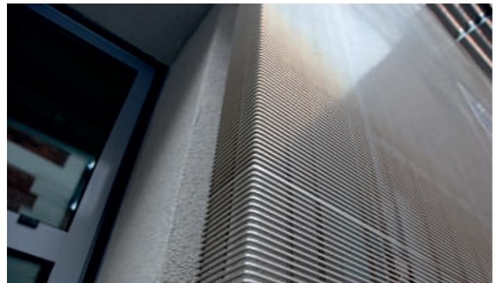
Facade grid bent in the vertical plane
