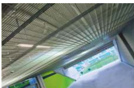
Stadium Wrocław / Wrocław
